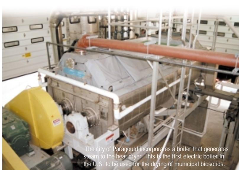
The city of Paragould incorporates a boiler that generates steam to the heat dryer. This is the first electric boiler in the U.S. to be used for the drying of municipal biosolids.
